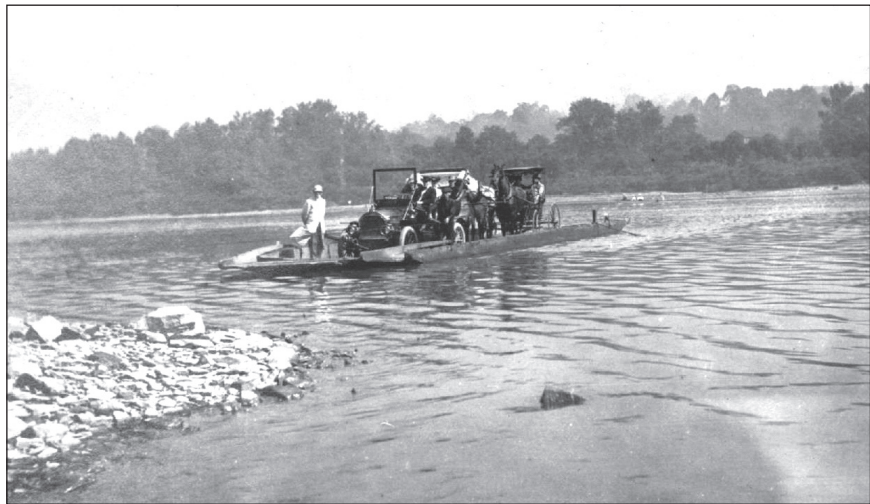
Before there was a Sewickley Bridge
