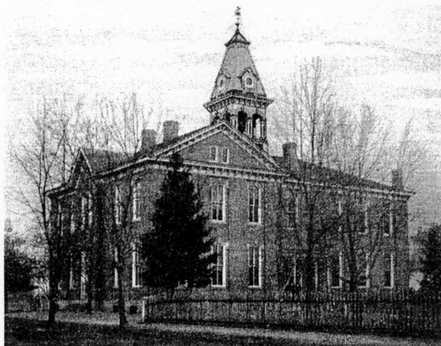
Sewickley Public School, destroyed by fire February 1, 1893. The first four rooms of the school were built in 1862, and eight more had been added by 1882. The school stood on the Thorn Street site of the "yellow brick school" designed by Elmer E. Miller in 1894 and razed in 1975.
